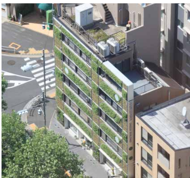
04: Two examples of buildings with green curtains in Tokyo, Japan. Photography by Meltem Senol Balaban and Raquel Moreno-Penaranda.
