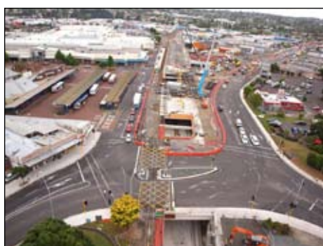
Overview of trench from western end
