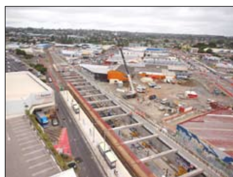
Overview of platform area from northern side
